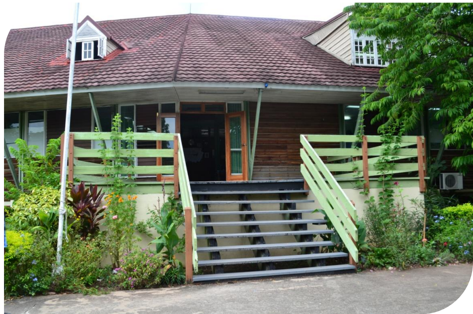
Forestry Department Head Office.
